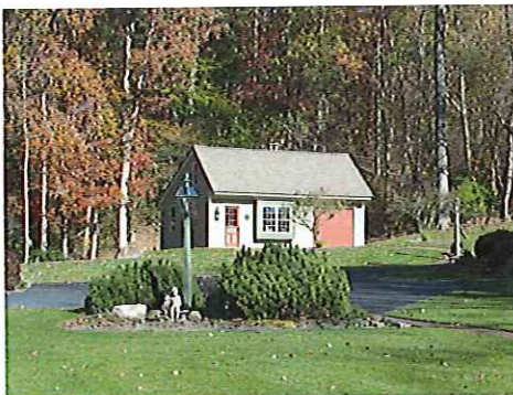
Wood Working Shop/Garage
